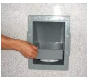
2. Ta ut filter locket
